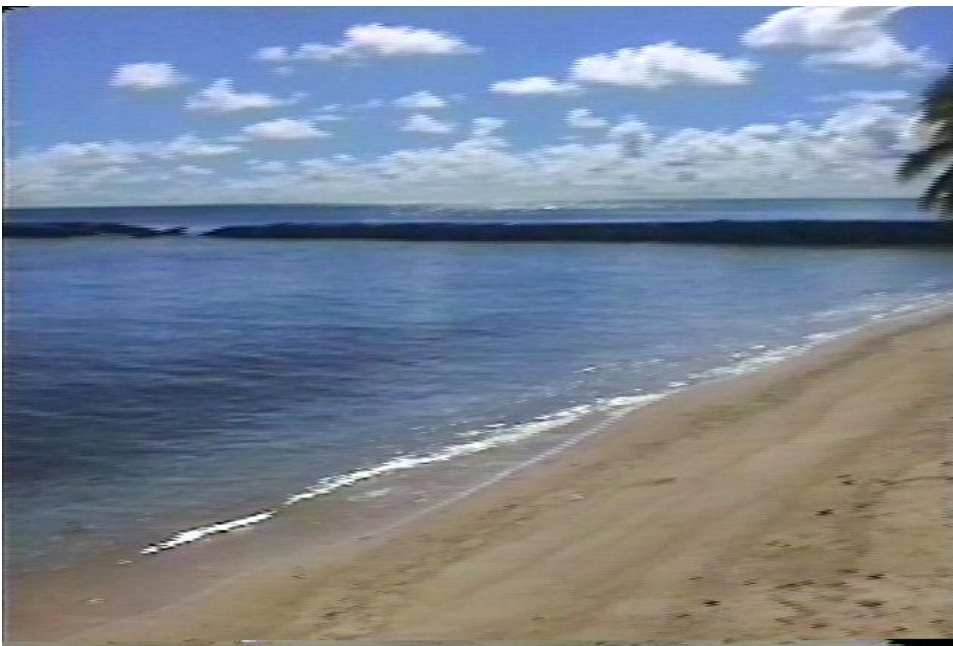
Site 6 Photo 3. The Japanese pier at Pigete Island from the south. Note the damaged section near the end, struck by American bombs during the war.
