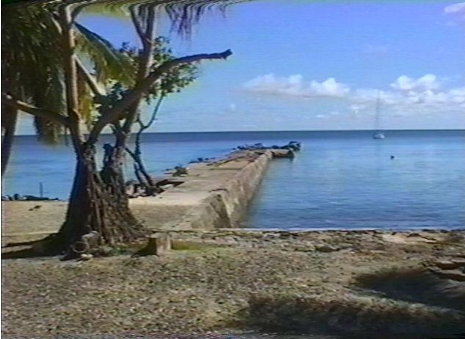
Site 6 Photo 2. The Japanese Pier at Pigete stretches nearly 100 yards from the natural shoreline. The pipe trench, blown open farther down on the right side, held both water and fuel lines. An anti-aircraft position was set up on the right side end.
