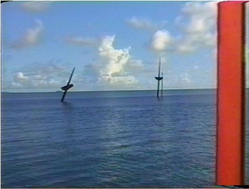
Site 8 Photo 1. The two main service masts still stand after 60 years in the water.
