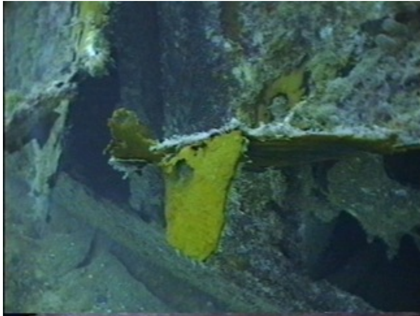
Photo KS4-7 Steel sheeting added to below the waterline . Note section fallen away at top left of photo which is next to the engine room.
