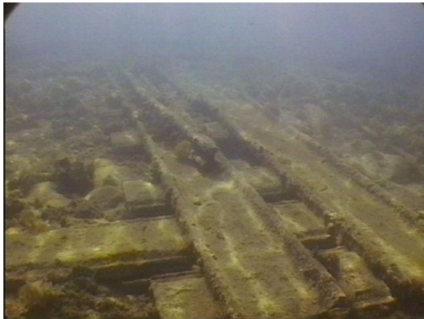
Photo MS7-3 The underwater section of Marine Railway, near end of southern segment.
