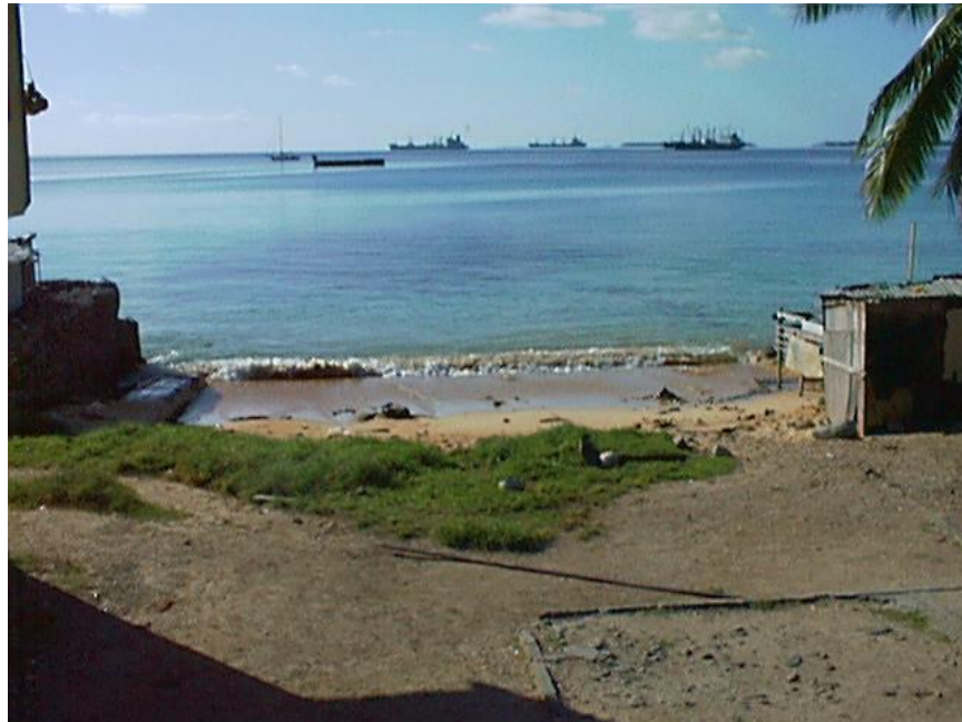
Photo MS8-1 Majuro Seaplane Ramp today. Concrete side rails in sand.
