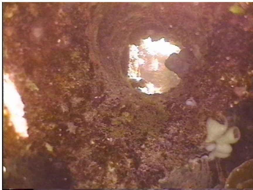
Photo MS4-6 Hole through concrete "Dead-man" where telephone pole was originally placed in concrete.
