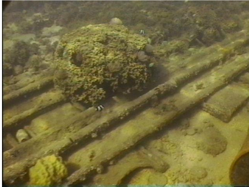
Photo MS7-4 Coral growth on Marine Railway. Sheet pile foundation can be easily seen, along with trash and debris, including a 55 gallon drum at right edge of the photo on the southern section of the railway.
