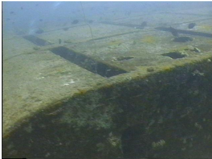
MS6-3 Floating barge section sunk off-shore of the 2 nd barge section in 30 feet of water.
