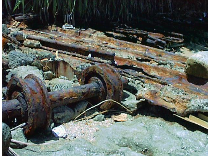
Photo MS7-2 Northern section of Marine Railway at tidal zone during low tide. The wheels are for original carriage to support hauled-out small craft.
