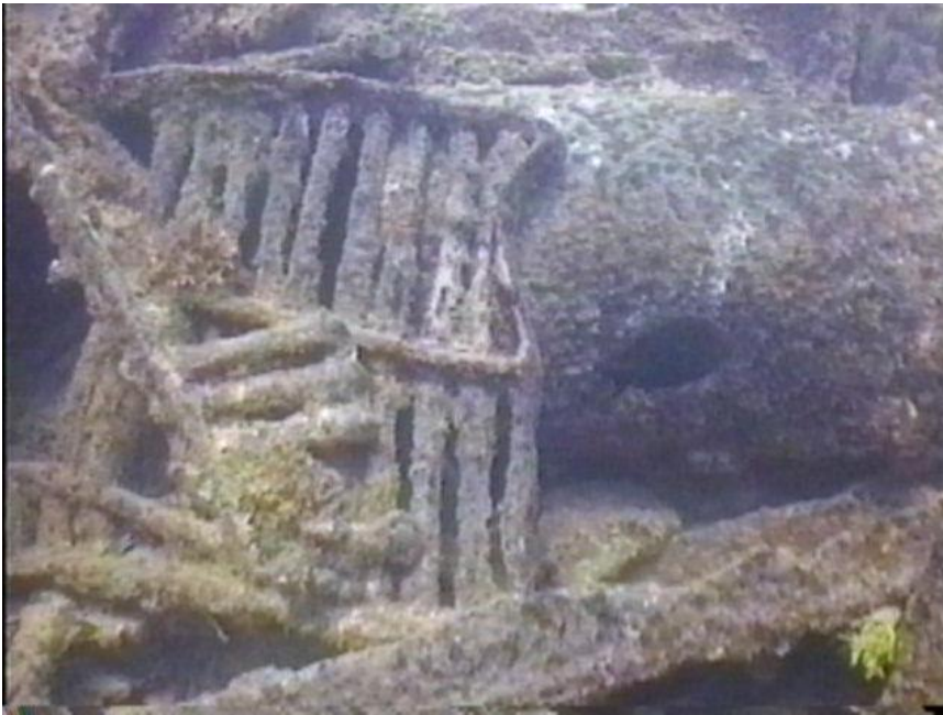
Photo Mi-9-8. A section of broken engine room catwalk near the boiler.
