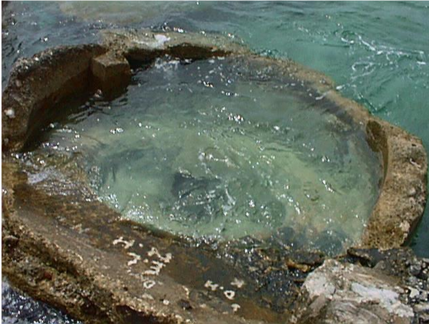
Photo WT6-4. Anti-Aircraft Site blown into water from bomb damage at the end of the Main Service Dock.
