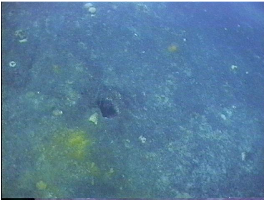
Photo WT12-17. Small hole in stern on starboard side, probably from Naval artillery shell.
