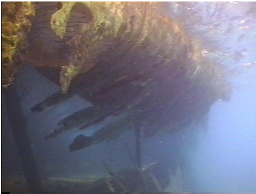
Photo WT13-6. Inside bow looking to starboard damage. This damage is probably from the weight of the bow crushing the underwater structure, but could also be from near bomb misses.
