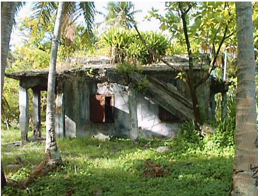
Photo WT4-7. Seaplane Operations Buildings, inshore from Seaplane Ramp.
