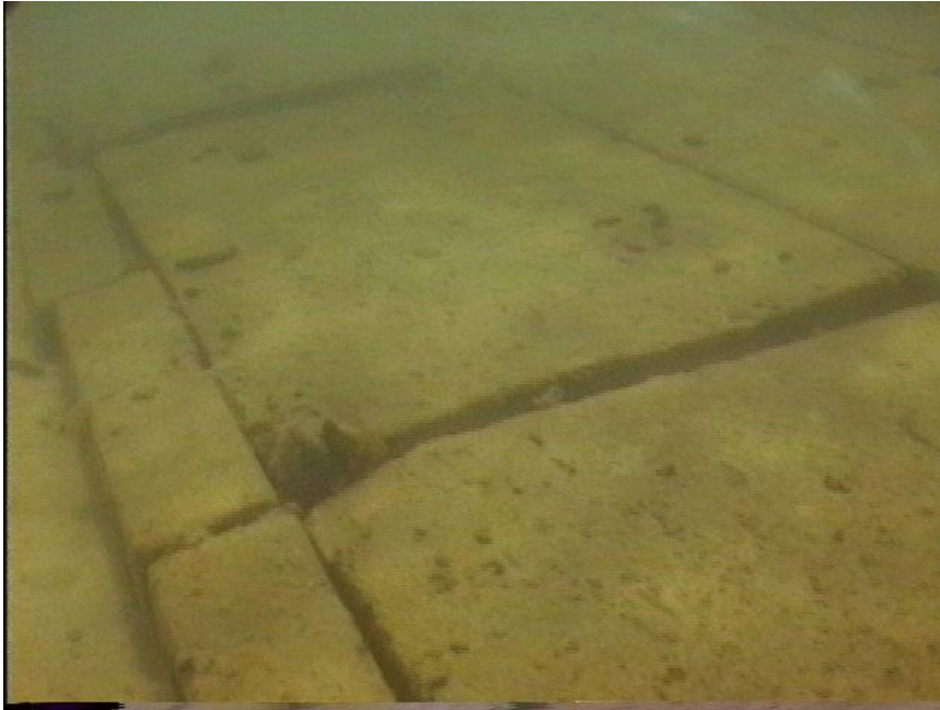
Photo WT4-2. Start of the ramp in deep water, south-west side.
