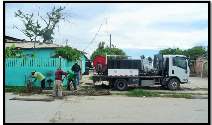
KAJUR Water & Sanitation Project Clearing Storm & Sewer Drains
